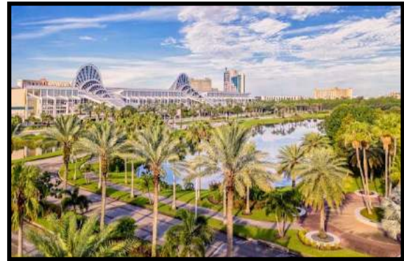
The OCCC North-South Building
